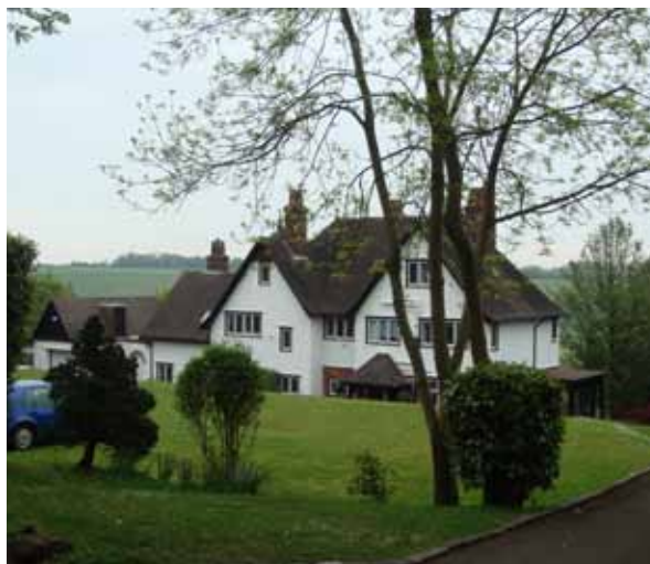
Figure 6.1: Examples of houses that are set below road level.
