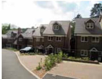
Figure 4.6: An example where the plots are not large enough to accommodate detached houses, leading to the loss of trees and vegetation. There is also not enough space for well integrated car parking resulting in the loss of front gardens.
