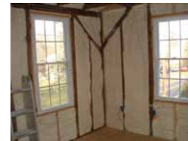
Figure 9.1: There are a number of techniques to improve the energy efficiency of existing buildings without destroying the appearance of it: Internal wall and loft insulation.
